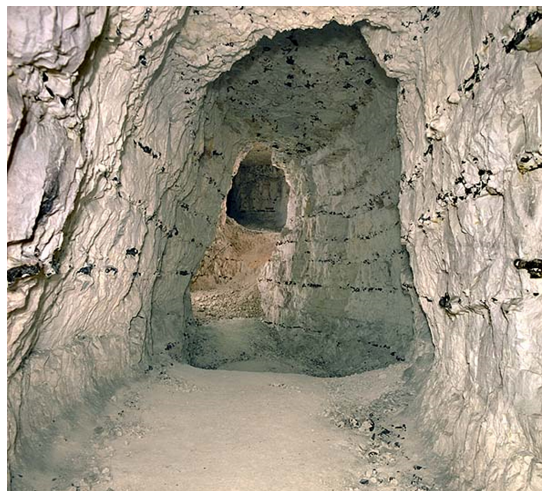
Fig. 6. Seaford Chalk Formation, Pinner Chalk mines, showing regular distribution of flint bands. Photo: Kirkman, K, 1992. Pinner Chalk Mines, Pinner Local History Society, with kind permission of the publishers.
