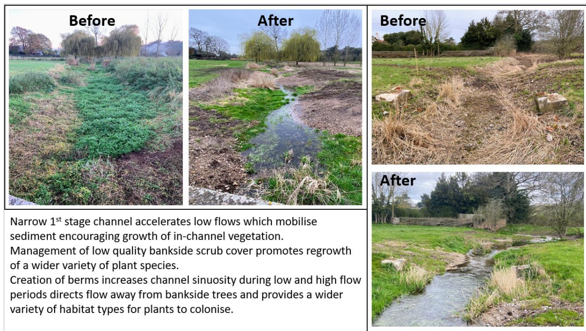
Figure 5: Hamble Brook channel restoration comparison
